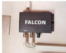
Tune TV 1 channel list for terrestrial TV then tune TV 2 again to terrestrial TV, if you see break up of picture then increase the strength on the booster by turning the strength control towards in the + direction.
