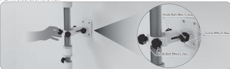
After adjusting azimuth, elevation and skew Fix bracket on the wall.
